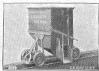
No. 0128 Generators Charging Car, Northern Gas Light Co., N. Y.
