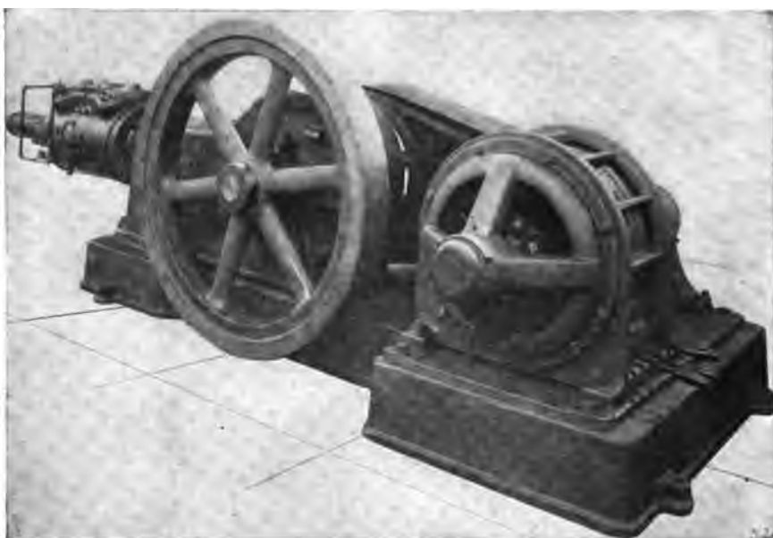
FIG. 28.—Ingersoll-Rand Compressor, Chain-Driven from an Electric Motor. Class "NE-1," 12\frac{1}{2} " \times 12" Cylinder.
