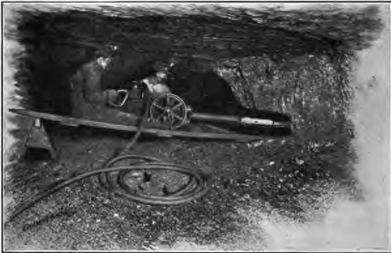
FIG. 199.—Sullivan Coal Pick, Working in a Thin Vein.
