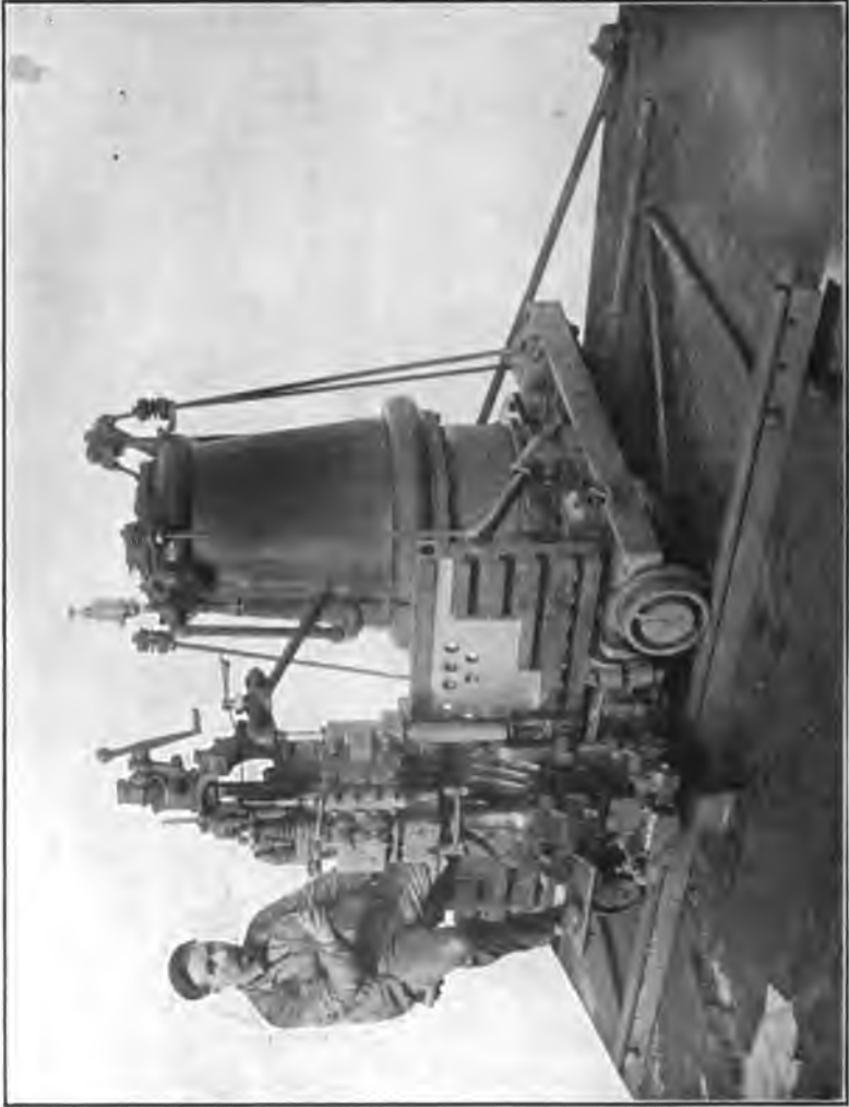
FIG. 212.—Ingersoll-Rand Ram Track Channeler, for Marble.
