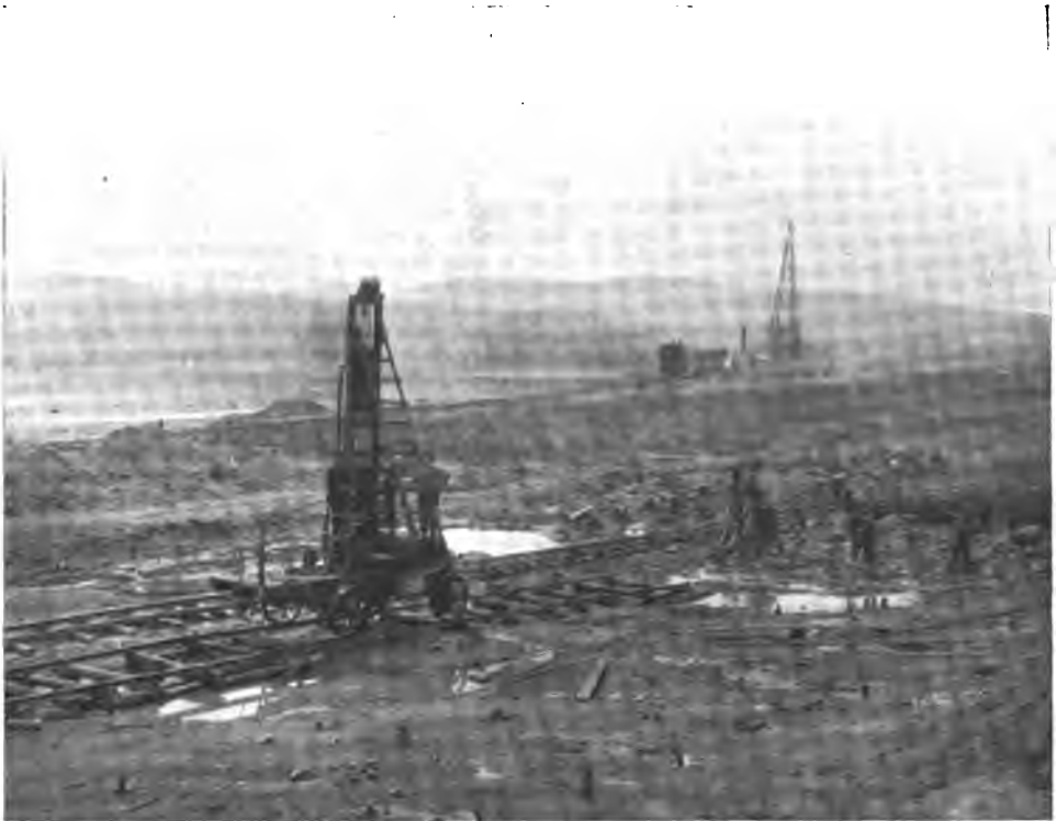
FIG. 1. GENERAL VIEW OF CHANNEL WORK IN THE HUDSON NEAR MECHANICVILLE.
