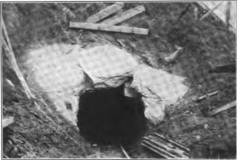
FIG. 3. MOUTH OF TUNNEL.
