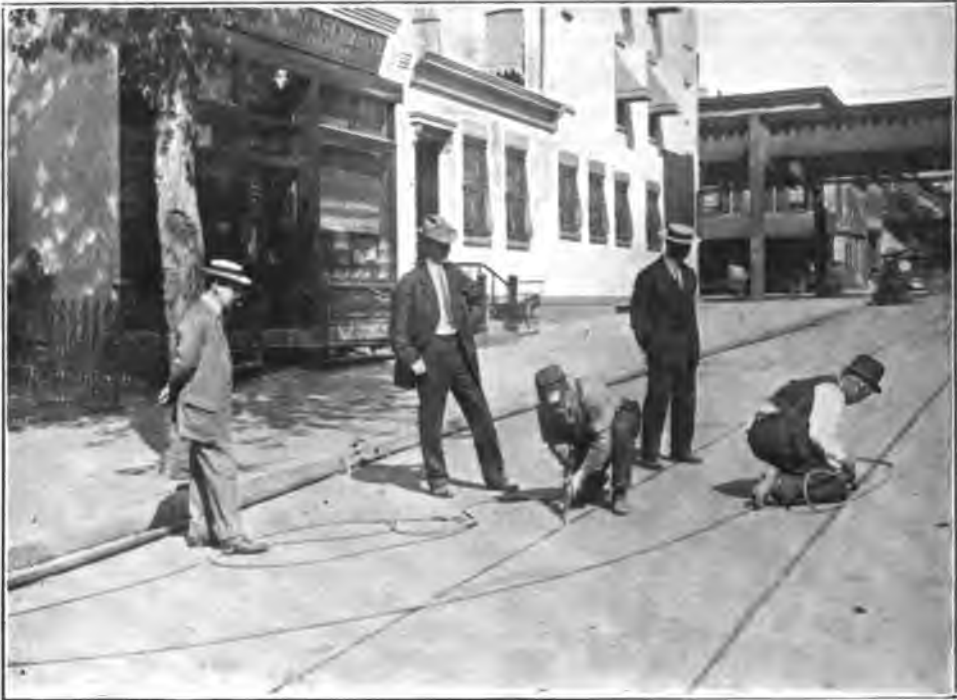
FIG. 3. CUTTING ASPHALT, BROOKLYN.
