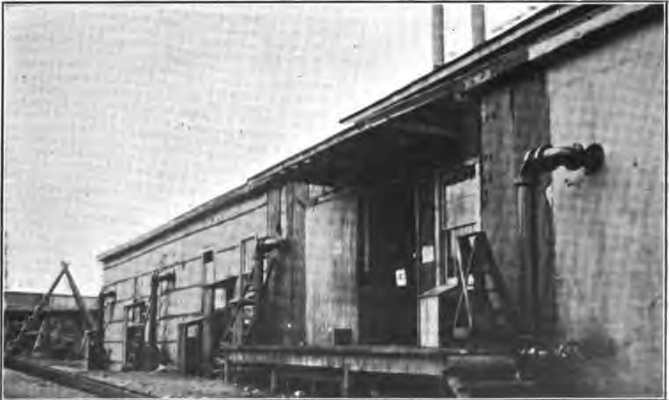
FIG. 4. INTAKE AND DELIVERY PIPES.
