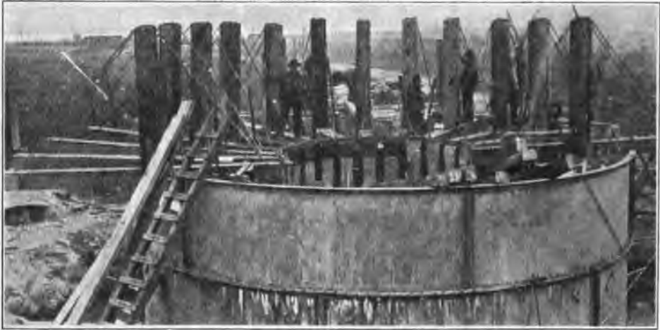
CANTILEVER FOR TRIMMING CAISSON.
