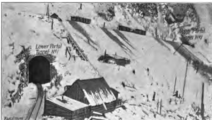
FIG. 1. BOTH PORTALS OF TUNNEL NO. 1.
