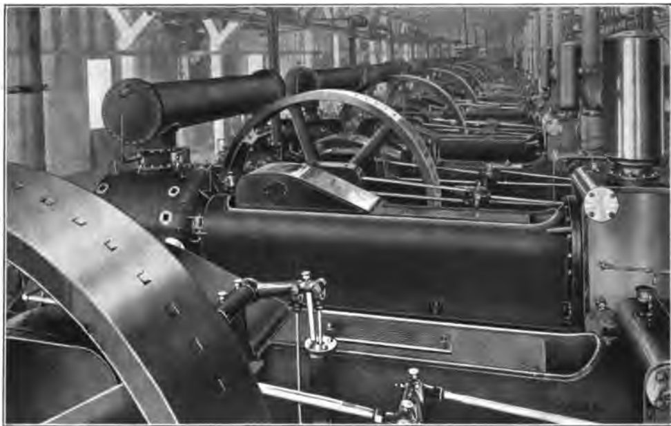
FIG. 2. INTERIOR OF COMPRESSOR HOUSE.
