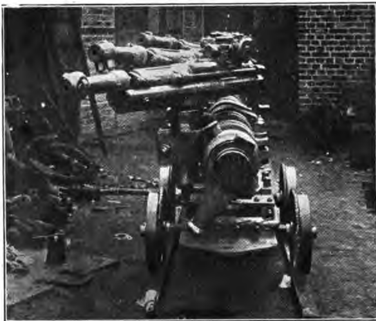
FIG. 1. CAR WITH DRILLS SWUNG AROUND TO RUN CAR BACK.
