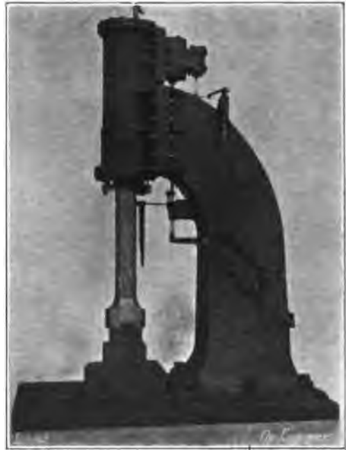
FIG. 7. HAMMER WITH EXPANSION VALVES
