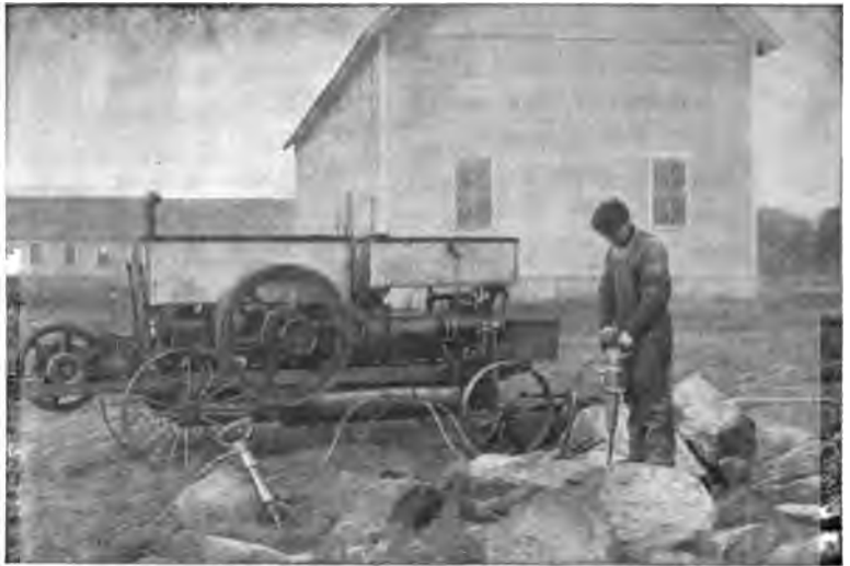
Sullivan "WK-3" Air Compressor Outfit and Sullivan "DB-15" Hammer Drills.
