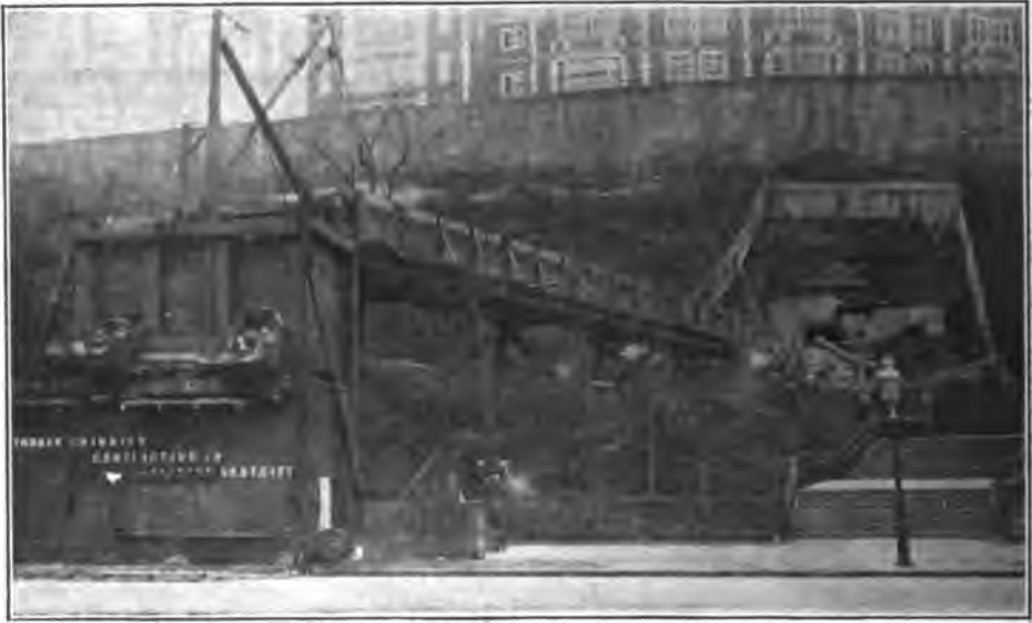
FIG. 2. COMPRESSOR HOUSE RUNWAY AND DUMP.
