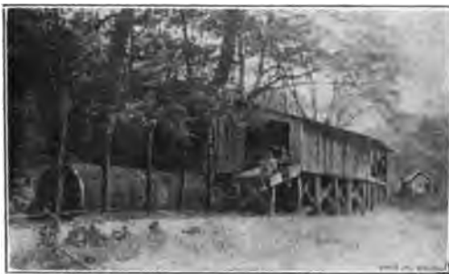
FIG. 3. STORAGE TANKS LOADING HOUSE AND MAG-NETO BUILDING.
