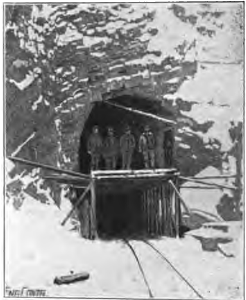
FIG. 4. UPPER PORTAL NO. 1 TUNNEL.
