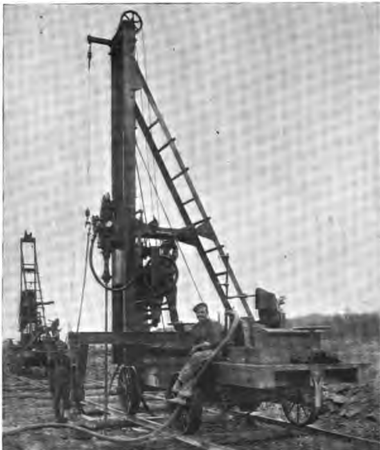
FIG. 2. TWO AUTOTRACTION DRILLS AT WORK.
