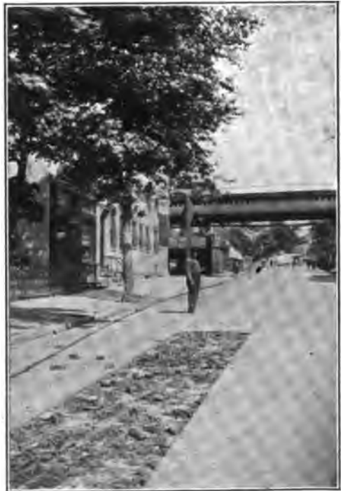
FIG. 5. READY TO DIG TRENCH.
