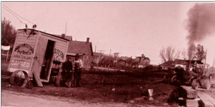
Emergency generation in Yankton during the 1930s was handled by a steam tractor-driven portable generator.
