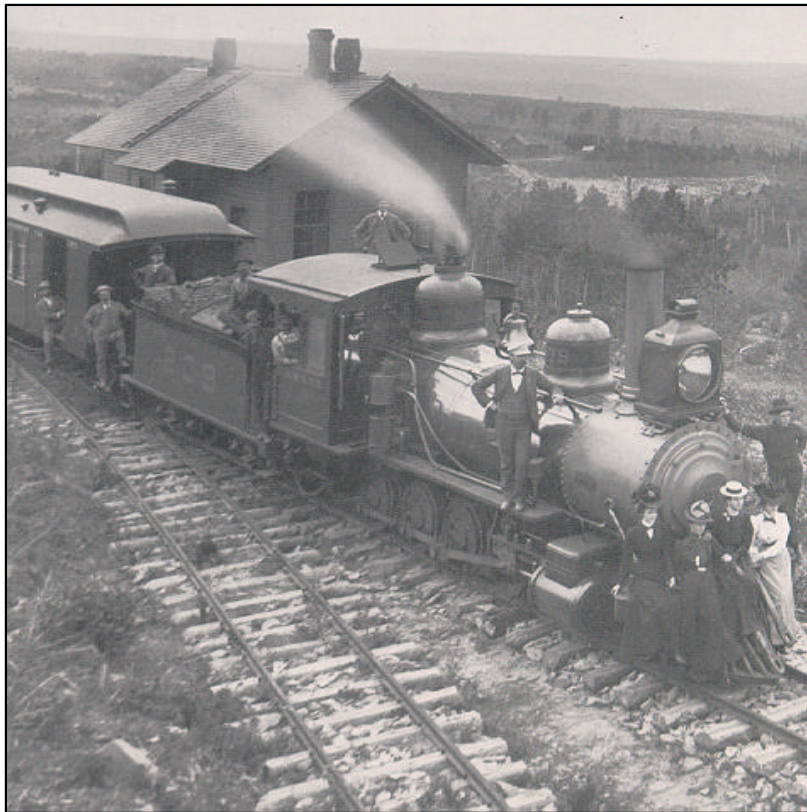
The “Cow Catcher” on the FE&MV Engine at the Crown Hill station holds a small group of ladies at the highest point on the line. The Elkhorn did limited passenger business concentrating on business with mines and small towns on the eastern side of Crown Hill.
